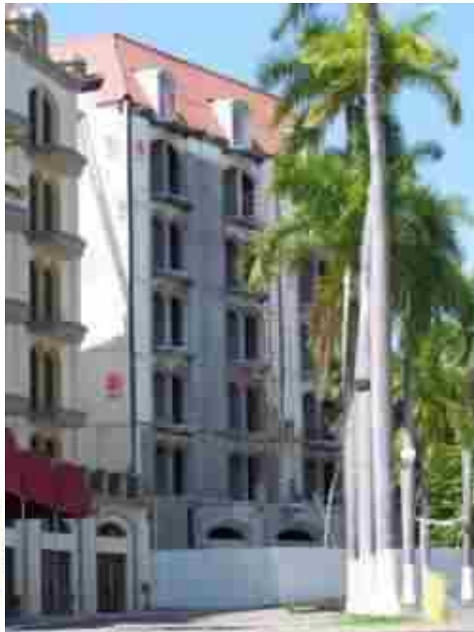
Panels integrated in STEEL STRUCTURE
